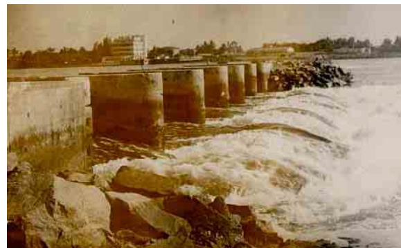
Figure 2.3 : Sluice dams at Cotonou channel mouth
