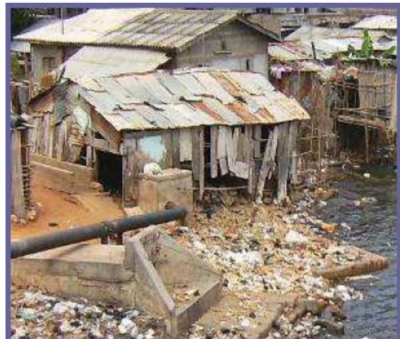
Figure 2.1 : outlet of rain waters or waste waters’ main sewer, drink water conduits stripped by erosion in an unhealthy environment on the banks of Cotonou lagoon
